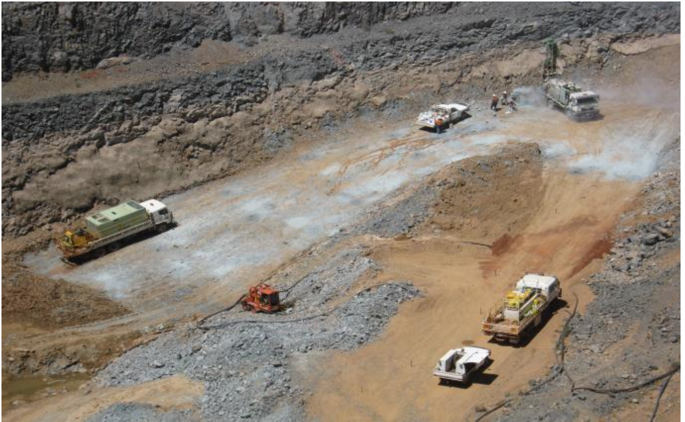
Figure 5. Previous resource drilling at the Celtic pit
